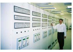
Figure 1. Alarm Annunciators in the power generation sector (Singapore).
